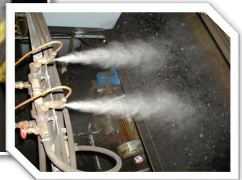
Extracting car, Trmice power plant Q = 500 t/h
