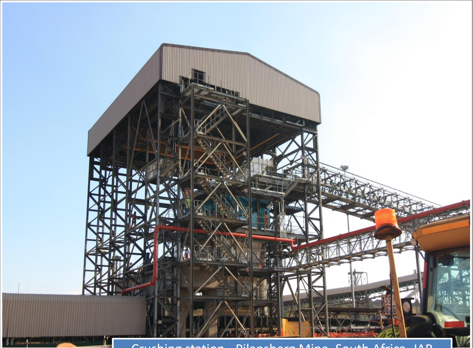
Crushing station - Pilansberg Mine, South Africa, JAR
