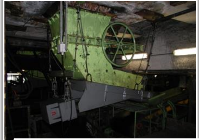
Vibrating feeder, Darkov Mine, OKD Q = 200 t/h
